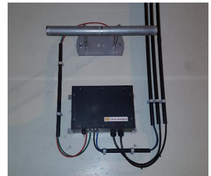
Pitot tube and terminal box Variant with differential pressure transducers in tunnel and one terminal box (pneumatic connection to both pitot tubes)
